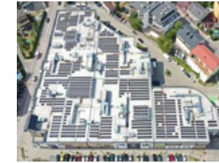
Project: Commercial PV Power System in Poland Location: Poland Capacity: 360kW Grid Connection Time: 2023.07
