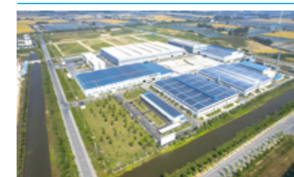
4.2MW Bosideng Logistic Zone PV Power Project
