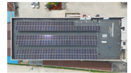
0.4MW Xinchangmaoye Rooftop PV Project
