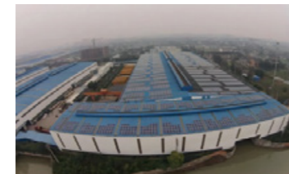
3.26MW Yulong Steel Factory Rooftop PV Project
