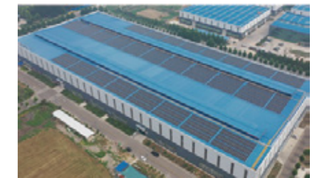
3.3MW Weike Group Rooftop PV Project
