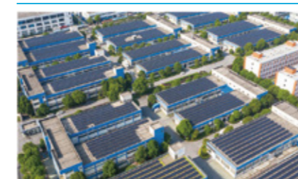
5.29MW Bosideng Comany PV Power Project
