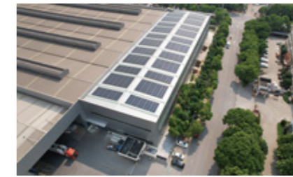
0.3MW Sunlit Factory Rooftop PV Project
